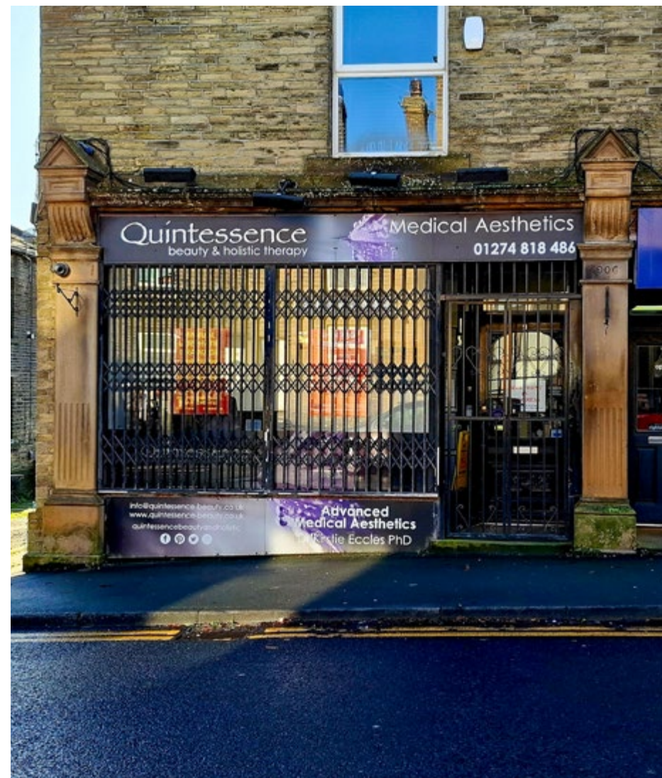
External security grills on a shopfront in Queensbury
