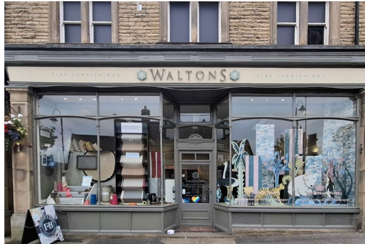
Waltons Fine Furnishings, Ilkley is a good example of a well preserved Edwardian shopfront
