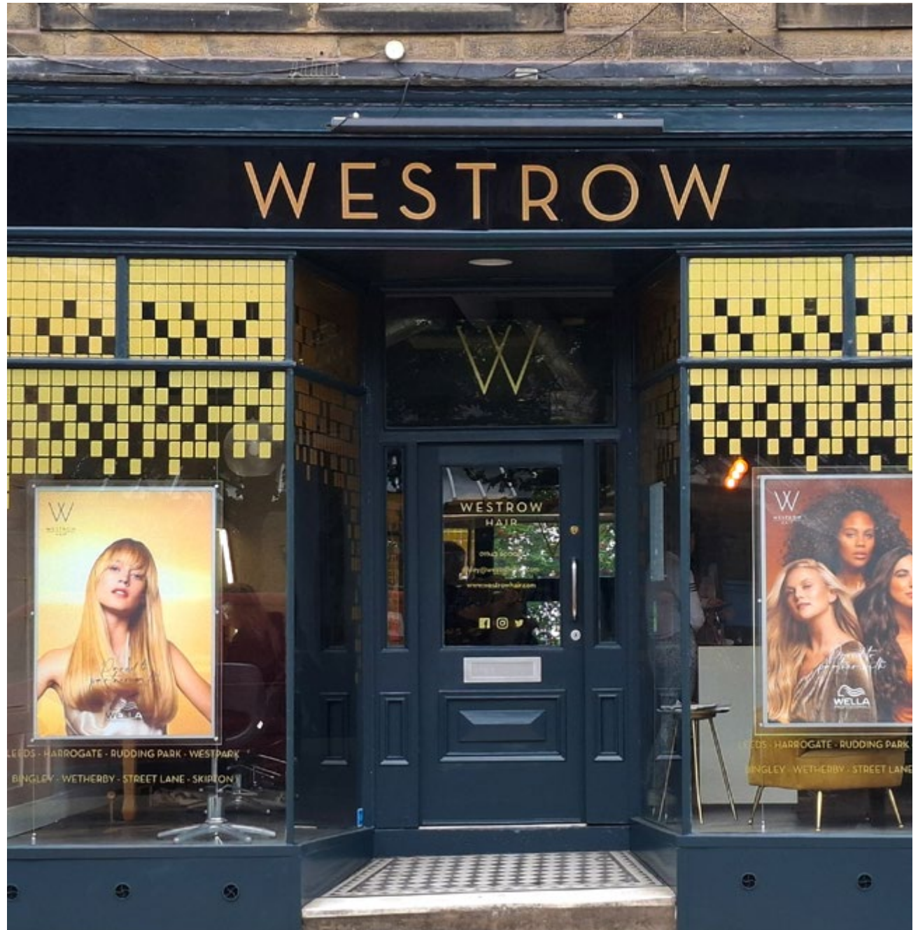
Stallriser ventilation on Westrow, Station Road, Ilkley
