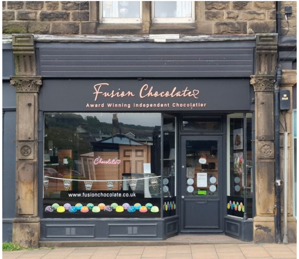
Well integrated ventilation in the stallriser of the shopfront, Fusion Chocolate, Leeds Rd, Ilkley
